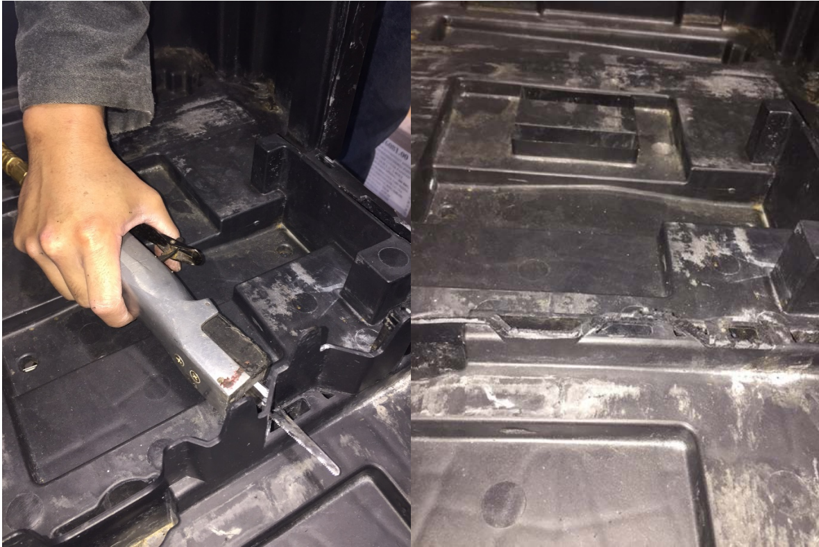
Fig. 6- Raised material removed.
