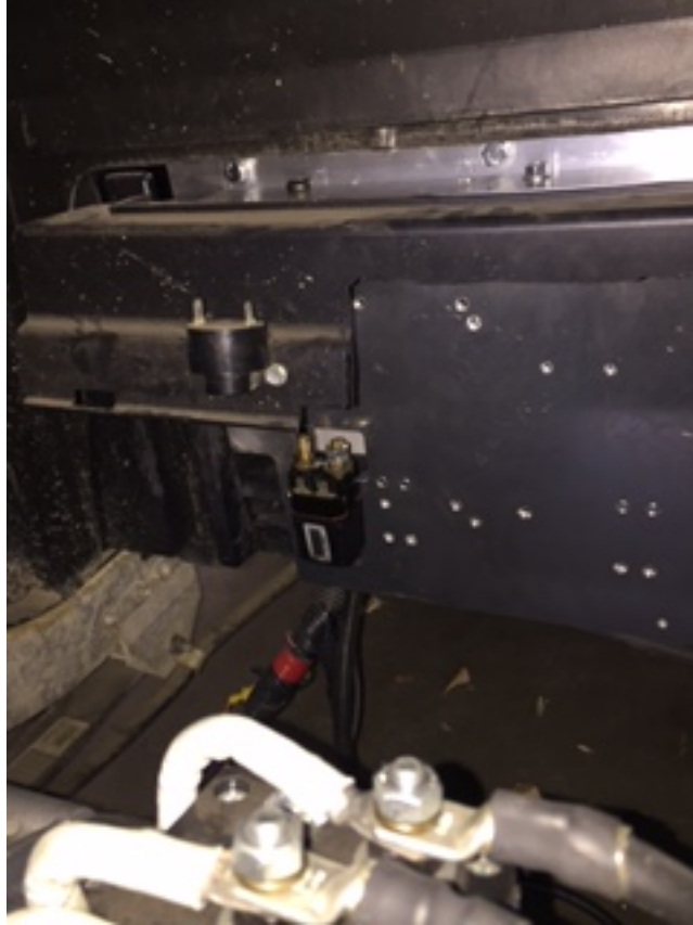
Fig. 20- Contactor installed on new controller plate
