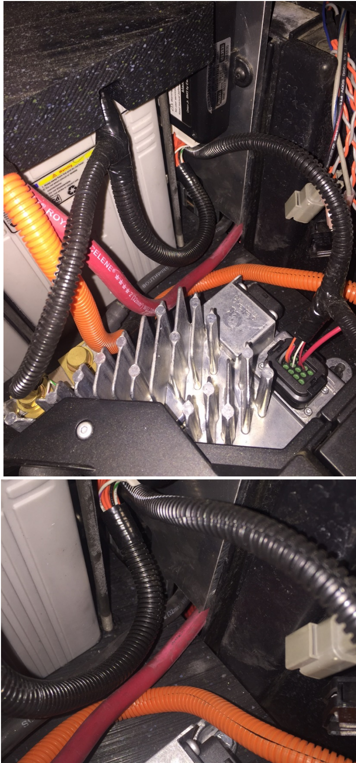
Fig. 23- Cable routing from battery pack
