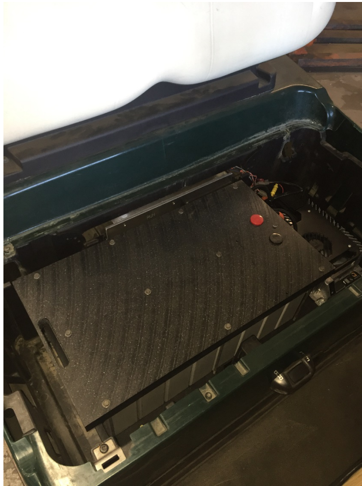
Fig. 11-Lithium battery pack installed into golf car
